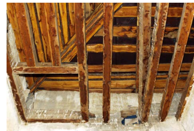
Ceiling at the west chamber where an opening was provided for climbing to an upper structure.
