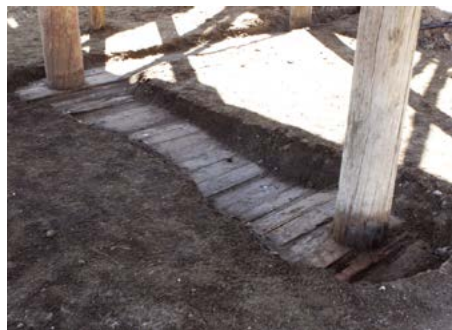
Trench in the floor for investigation
