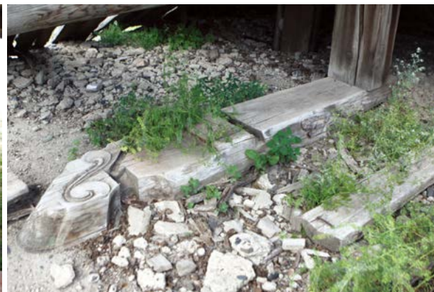
Beam wood used as bolster
