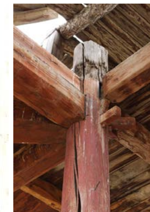
Joining part of an inner column
