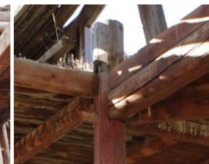
Joining top of the inner column
