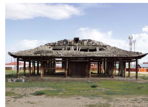
Front (south) view
