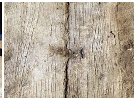
Connection with a damp rail
